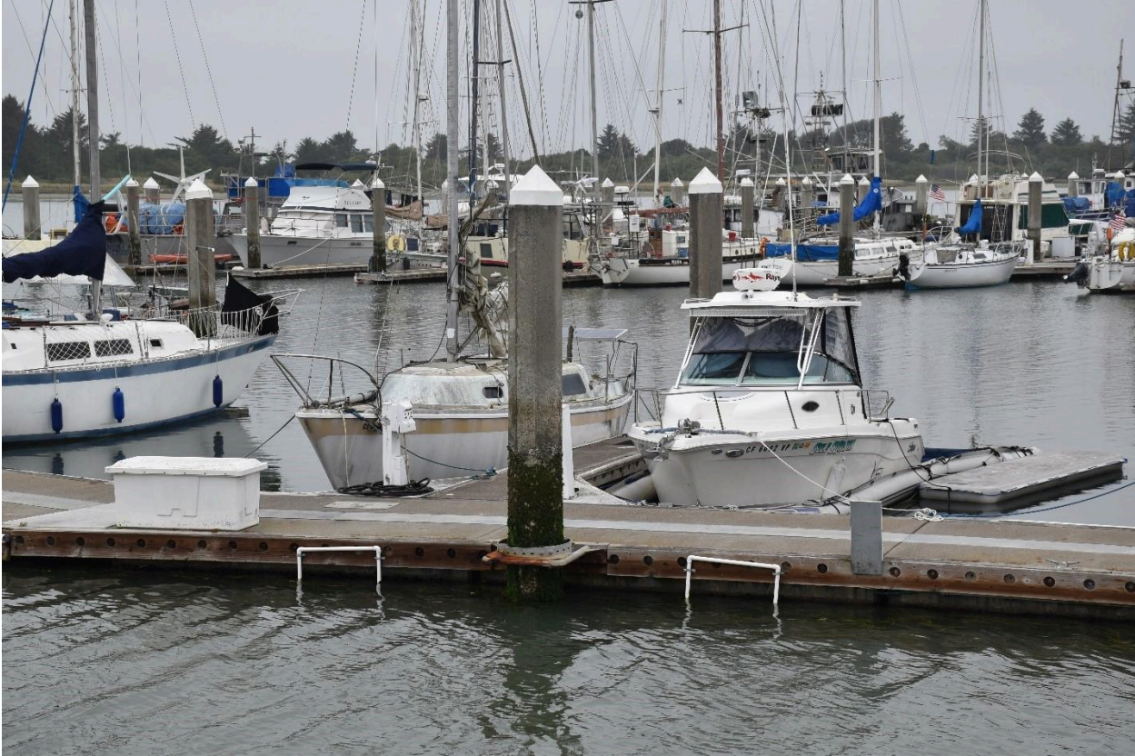
Figure 2. This image shows the placement of pallets 1 and 2 at the Eureka Public Marina (EPM). The pallets were placed on either side of the 5 th piling. They were fastened to the docks using pipe holders and 2” stainless steel screws.
